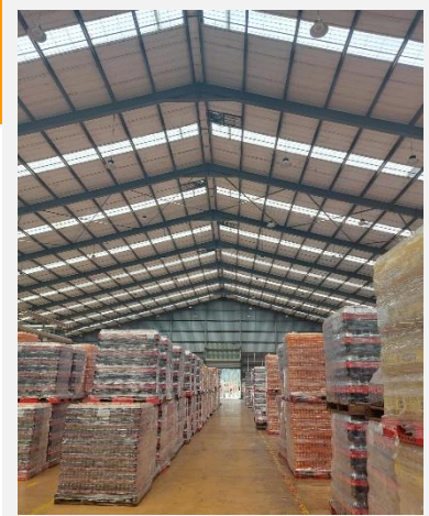
■ New natural skylights and LED installations provide a cost-saving lighting solution
